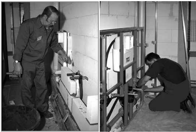
Brick-wall construction (left) versus dry-wall construction
