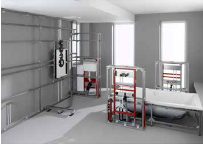
Bathroom walls with TECEprofil – before
